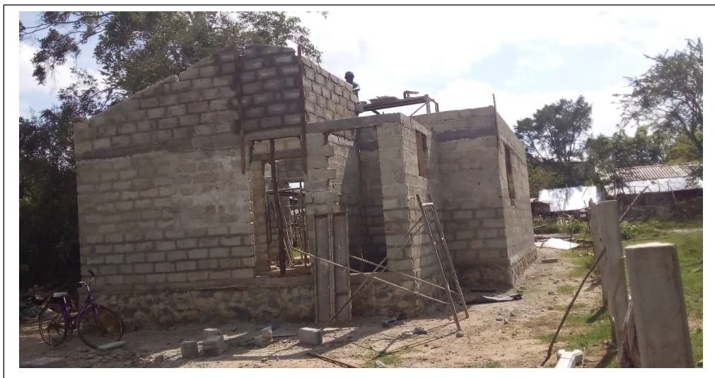
Progress Photos 3 (as on 30 Sep 2021)
