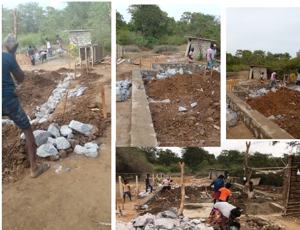
Progress Photos 2 (Foundation works)
