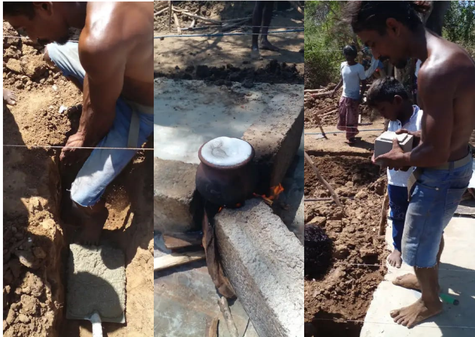
Progress Photos 1 (Day-1)
